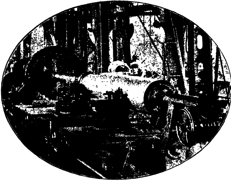
ROUGH-TURNING A GUN-BARREL IN TURNING MACHINE
